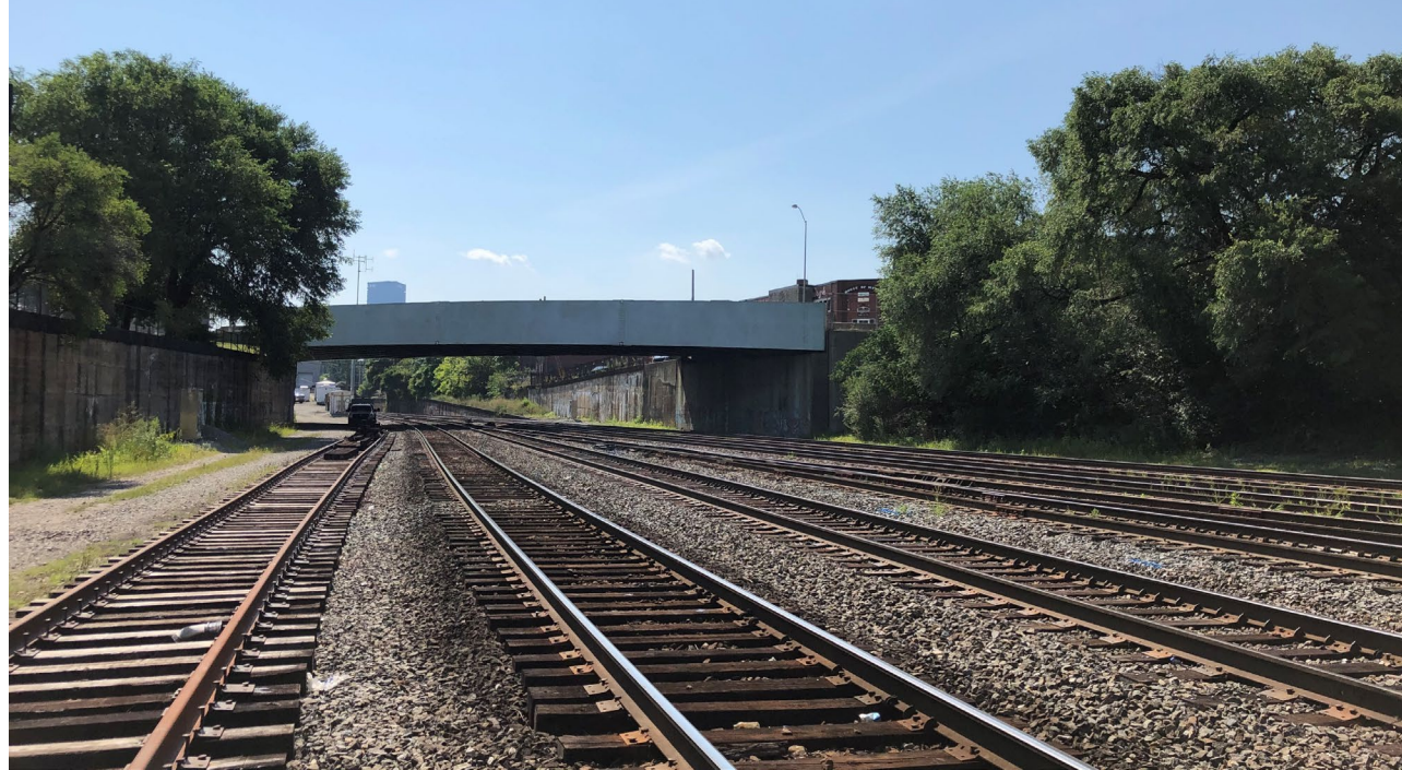
Photo of existing Pennsylvania Avenue Bridge, facing southwest.
