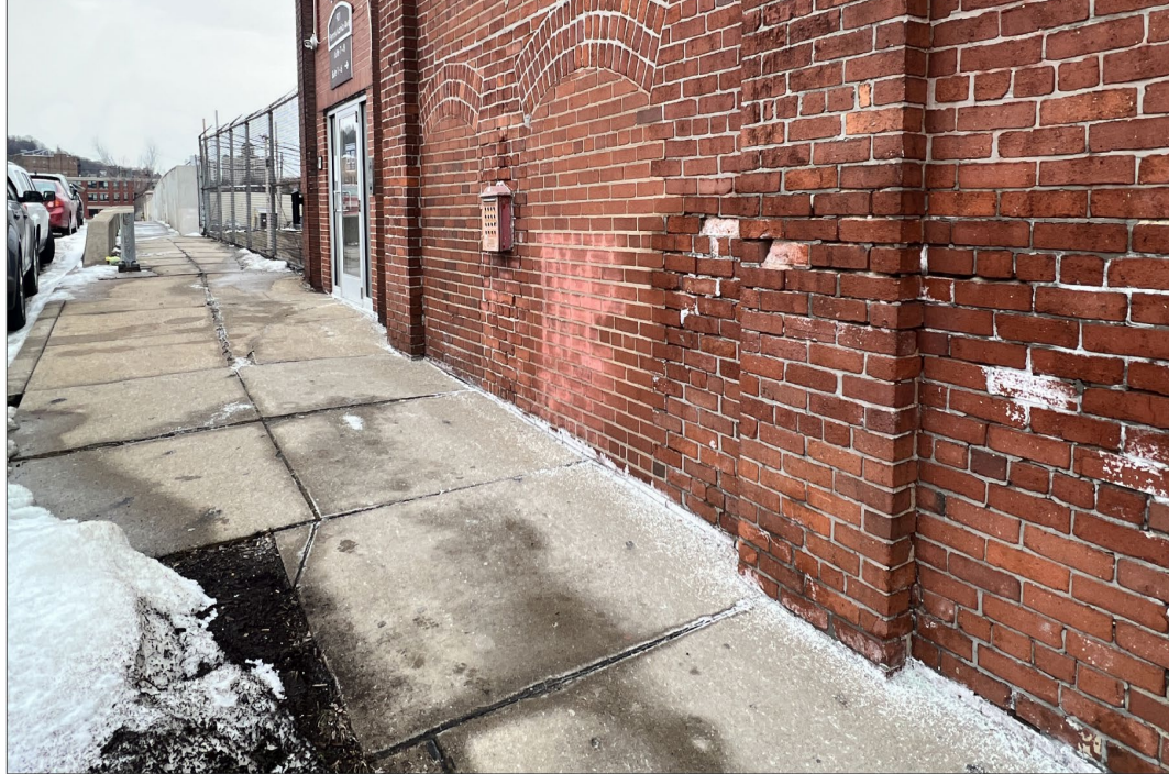
Photo of existing sidewalk and entrance to 901 Pennsylvania Avenue, facing southeast.
