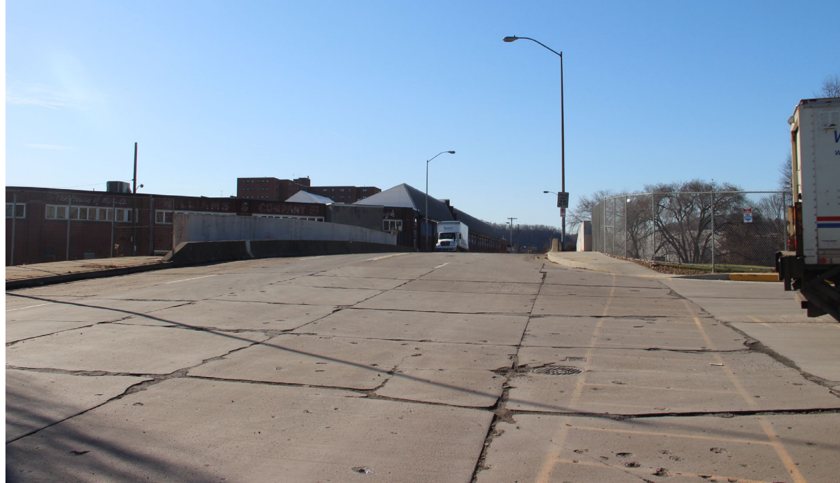
Photo of existing Pennsylvania Avenue Bridge, facing southwest.
