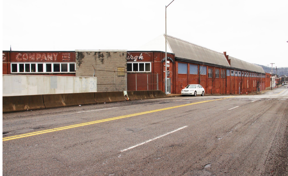
Photo of existing Pennsylvania Avenue Bridge, facing southwest.
