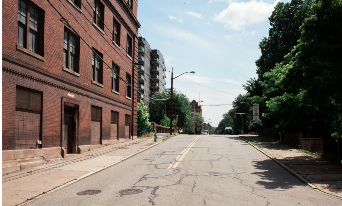
Photo of existing W. North Avenue Bridge from W. North Avenue, facing northeast.
