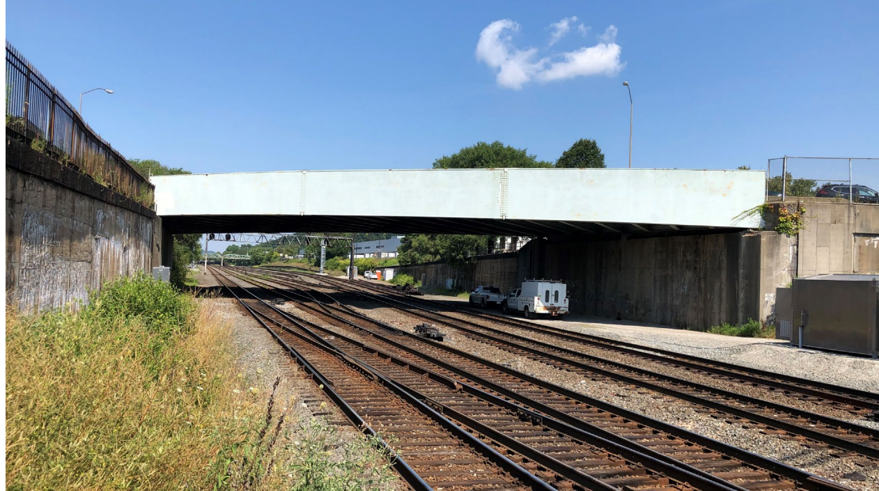
Photo of existing Pennsylvania Avenue Bridge, facing northwest.
