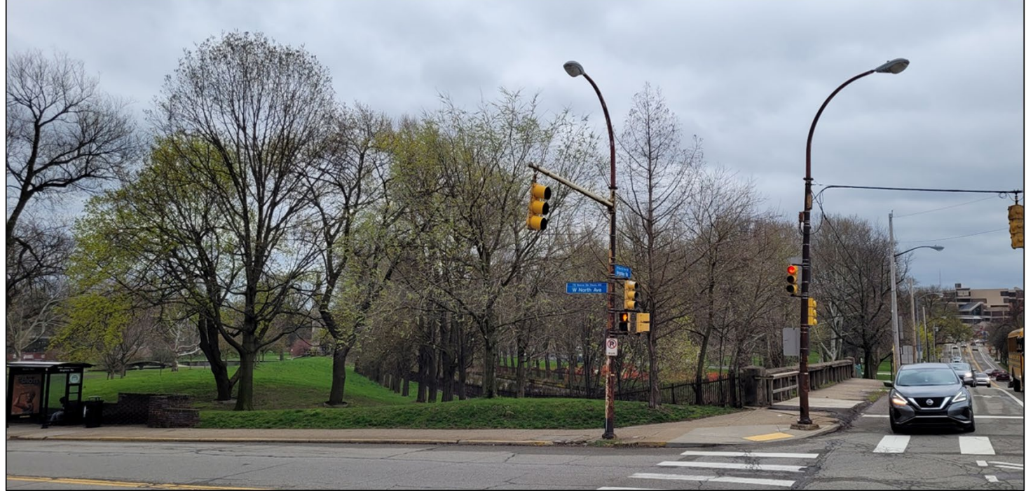
Photo of existing W. North Avenue Bridge from street level at the northeast corner of W. North Avenue and Brighton Road, facing southeast.
