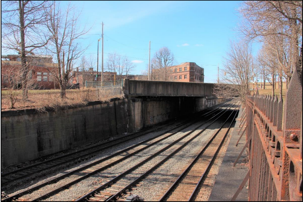
Figure 5-2: View of surveyed segment of rail corridor from Allegheny Commons Historic District showing the southeast side of the W. North Avenue Bridge, the southwest concrete retaining walls with stone coping, and decorative wrought iron fencing, facing west.
