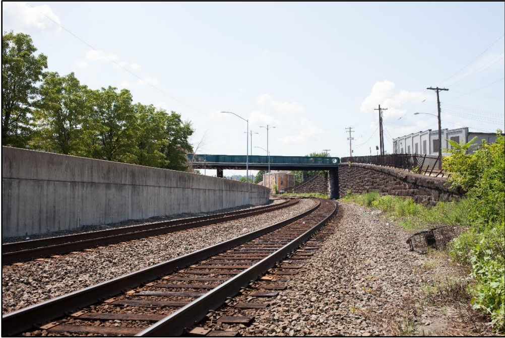
Figure 3-9: Photo of existing tracks under the Washington Avenue Bridge, facing south.
