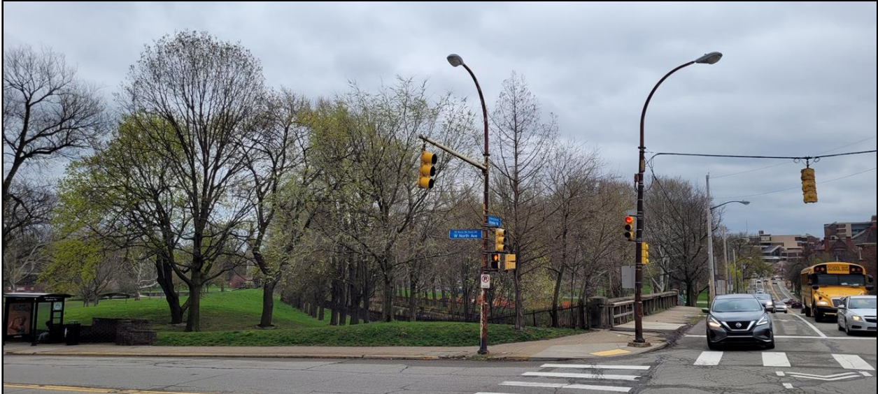
Figure 5-39: Photo of existing W. North Avenue Bridge from street level at the northeast corner of W. North Avenue and Brighton Road street level, facing southeast.
