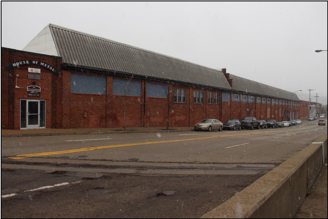
Figure 6-13: 901 Pennsylvania Avenue from the deck of the Pennsylvania Avenue Bridge, facing southwest.
