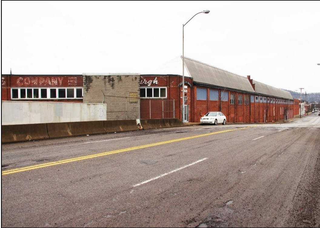
Figure 6-23: Photo of existing Pennsylvania Avenue Bridge from bridge deck showing 901 Pennsylvania Avenue, facing southwest.
