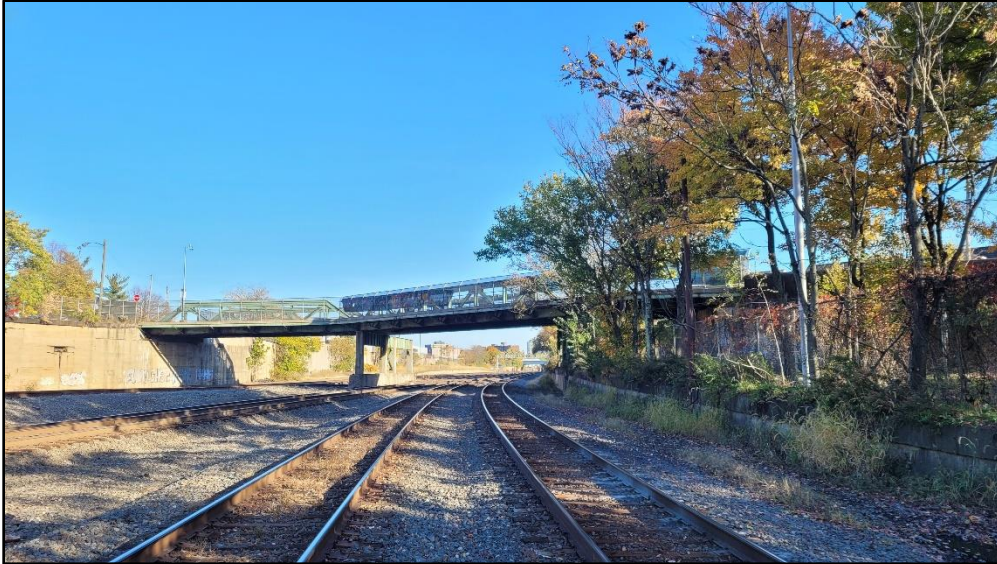
Figure 7-18: Photo of existing western-most main line tracks under the Columbus Avenue Bridge, facing southeast.
