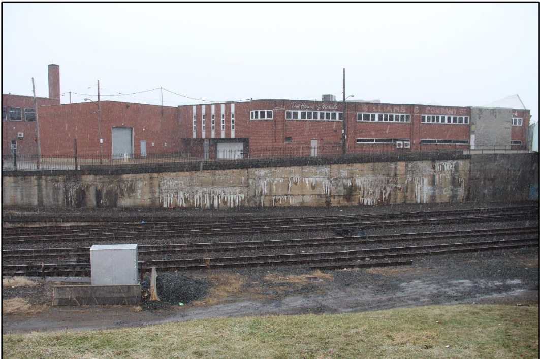
Figure 6-4: Concrete retaining walls with stone coping and decorative wrought iron fencing along the southwest side of the corridor and southeast of the Pennsylvania Avenue Bridge, facing southwest.
