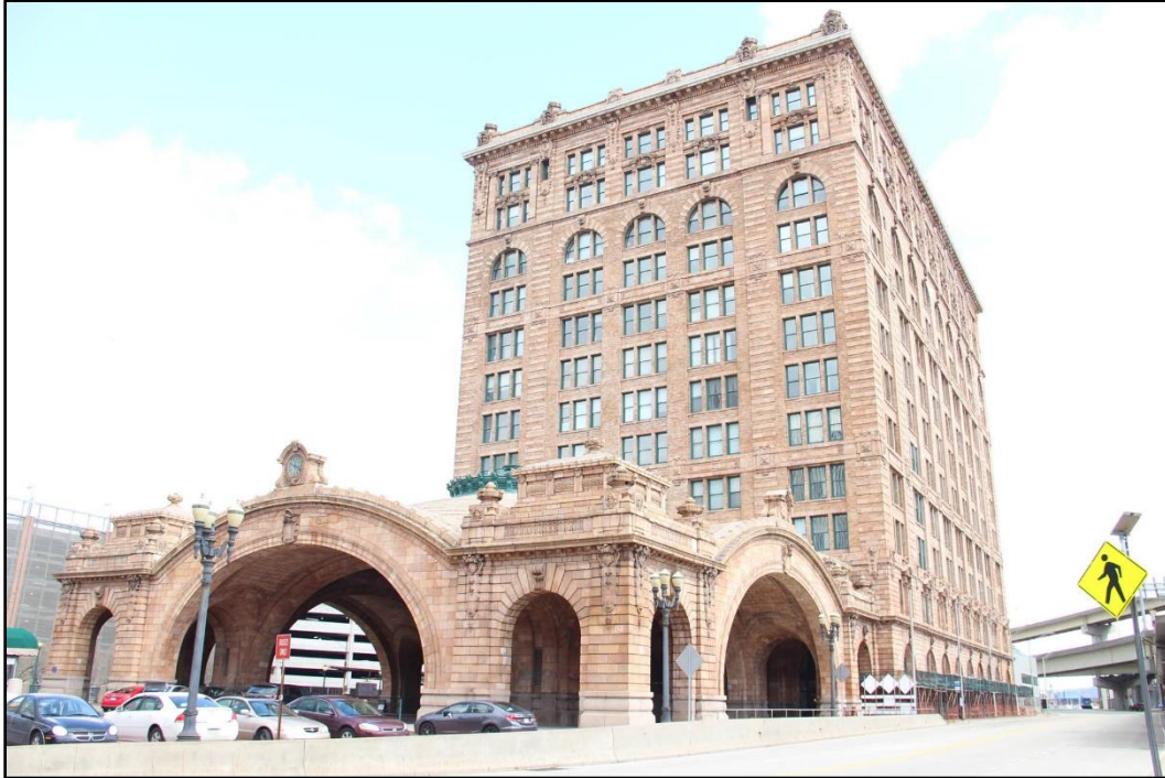
Figure 4-2: Overview, Pennsylvania Station (1900-03) showing station building and contributing rotunda. View from service drive and Martin Luther King, Jr. East Busway, facing north.
