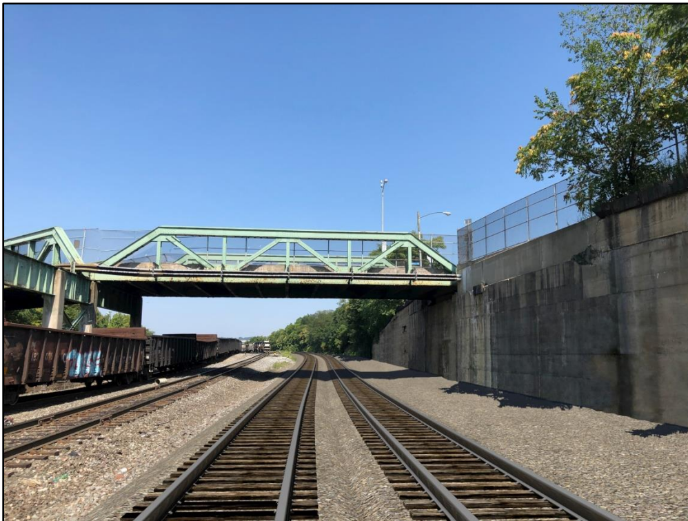
Figure 7-13: Rendering of lowered eastern-most main line tracks (Alternative 3A) under the Columbus Avenue Bridge, facing northwest.
