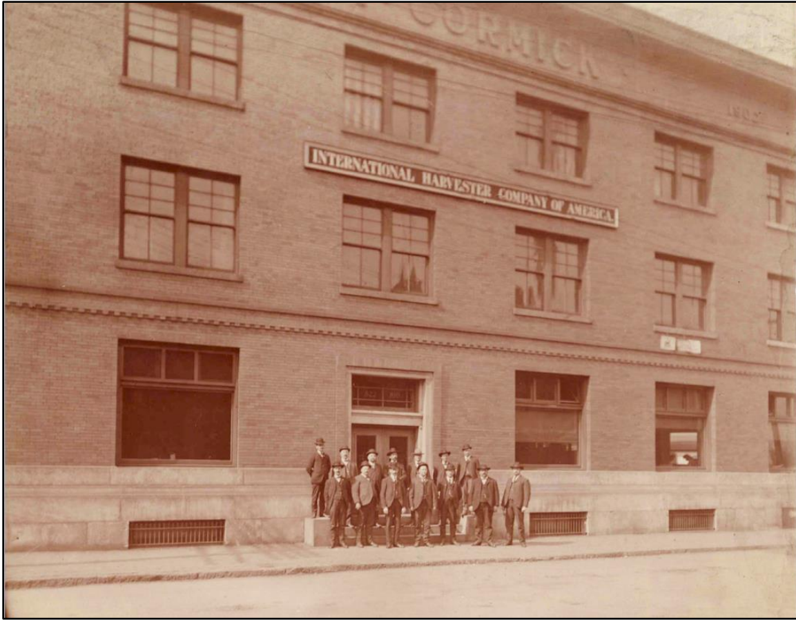
Figure 5-54: View of the International Harvester Building in 1904 showing the limestone foundation/water table and first floor windowsills prior to the grade separation of W. North Avenue and the rail corridor that occurred ca. 1906.
