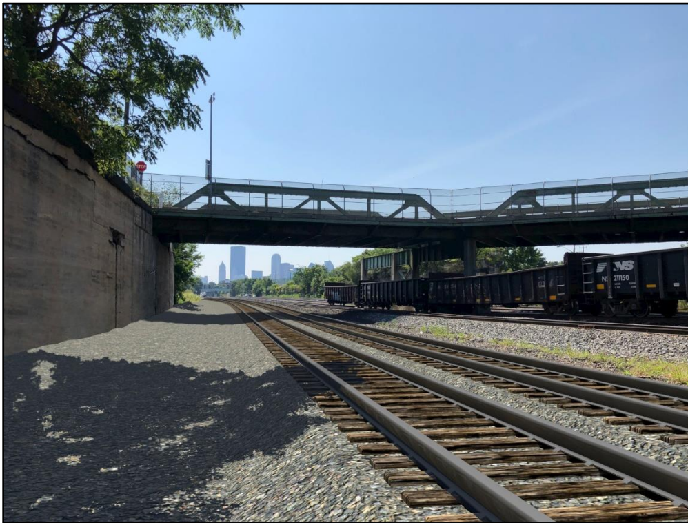
Figure 7-15: Rendering of lowered eastern-most main line tracks (Alternative 3A) under the Columbus Avenue Bridge, facing southeast.
