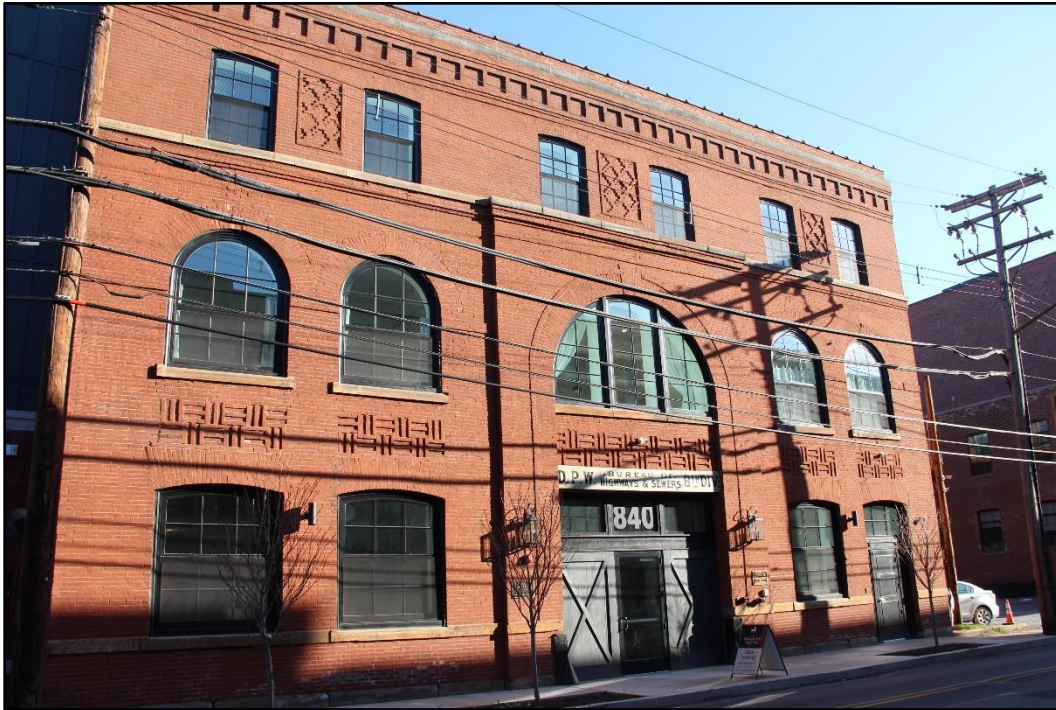
Figure 5-31: South (front) façade of the Allegheny City Stables Building at 840 W. North Avenue, facing northwest.
