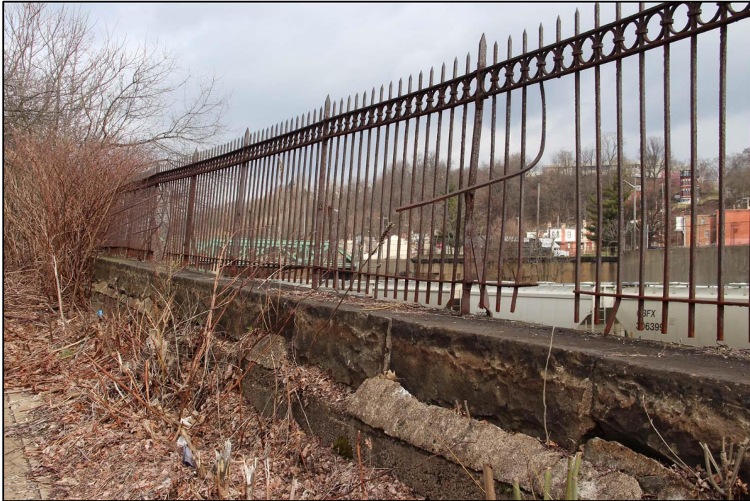
Figure 7-6: Detail of stone-capped retaining wall with wrought-iron fencing along northeast side of Allegheny Avenue, facing northwest.
