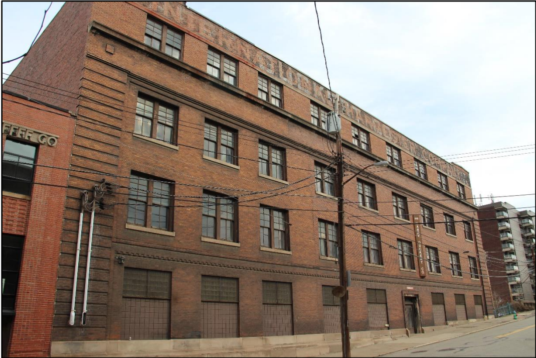
Figure 5-56: Current view of the International Harvester Building showing the stepped limestone foundation/water table and first floor windowsills of the three easternmost first-floor display windows after alterations from street grade changes ca. 1929 and again in the 1940s.
