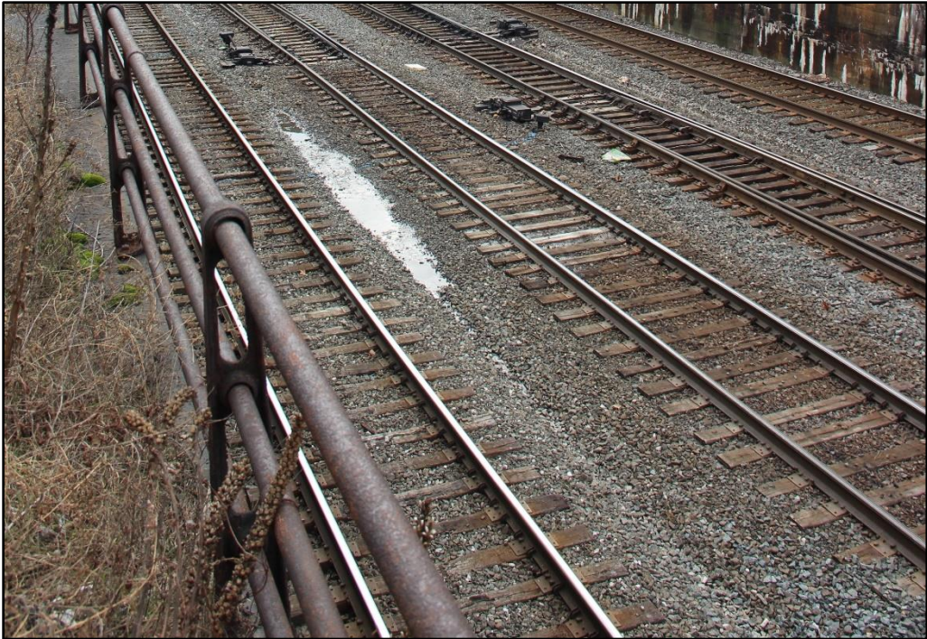
Figure 5-10: Detail of standard railroad safety fencing (left) atop edge of former elevated siding along the northeast side of the corridor north of the W. North Avenue Bridge, facing southeast.
