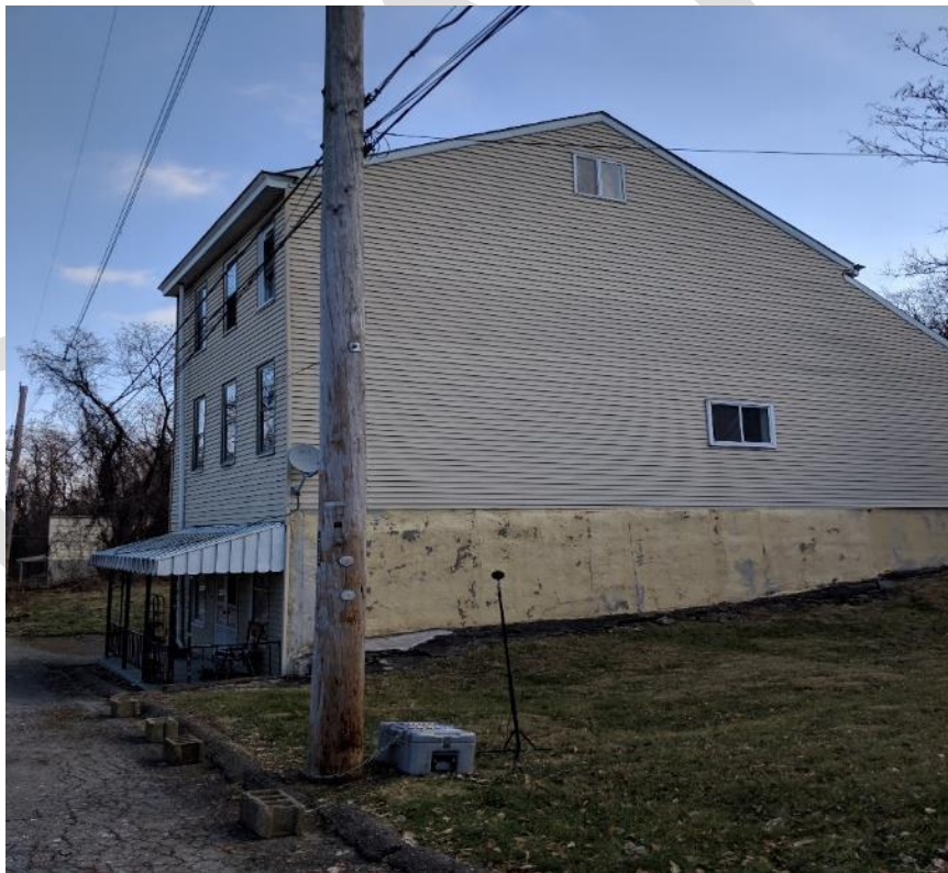
Figure A-10. Site LT-10: 2630 Brereton Street
