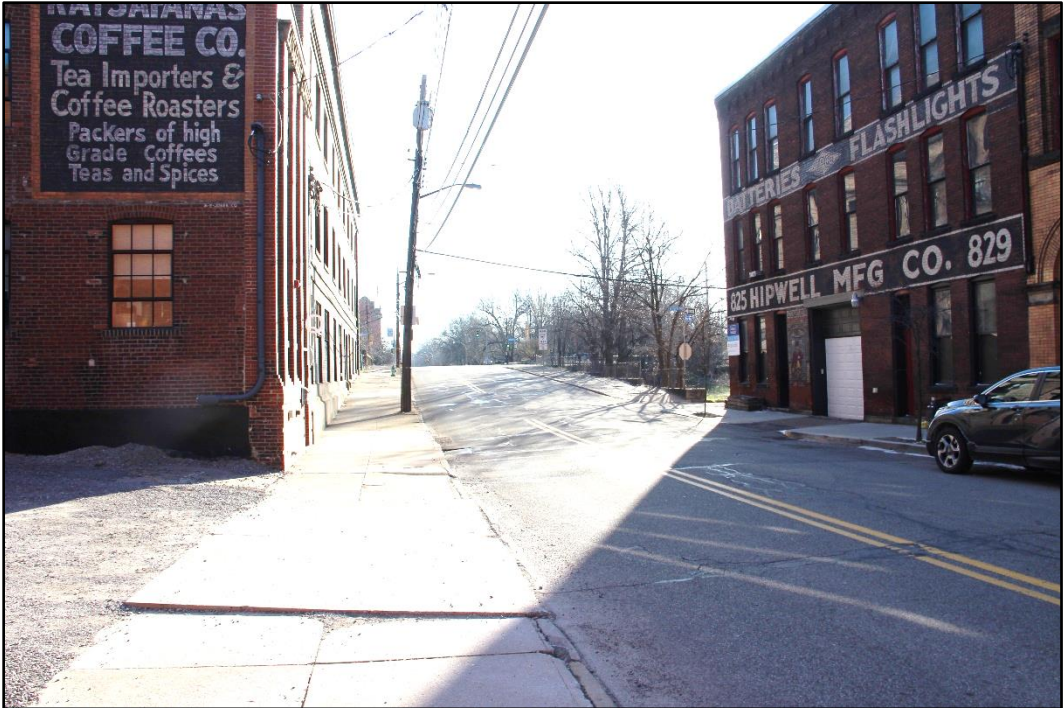
Figure 5-57: View from southeast corner of the Allegheny City Stables boundary along W. North Avenue, facing east. The vertical alignment adjustment in the 800 block of W. North Avenue would begin approximately 100' to the east.
