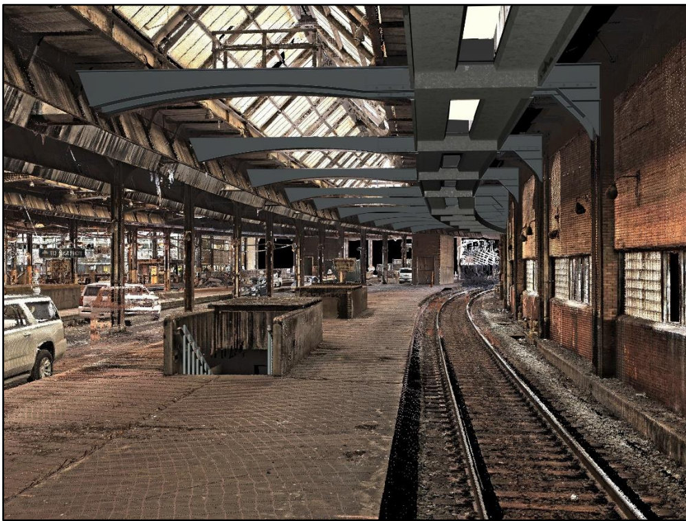
Figure 4-22: Rendering of retrofitted girders and exhaust chutes over Track 2 through trainshed, facing west.
