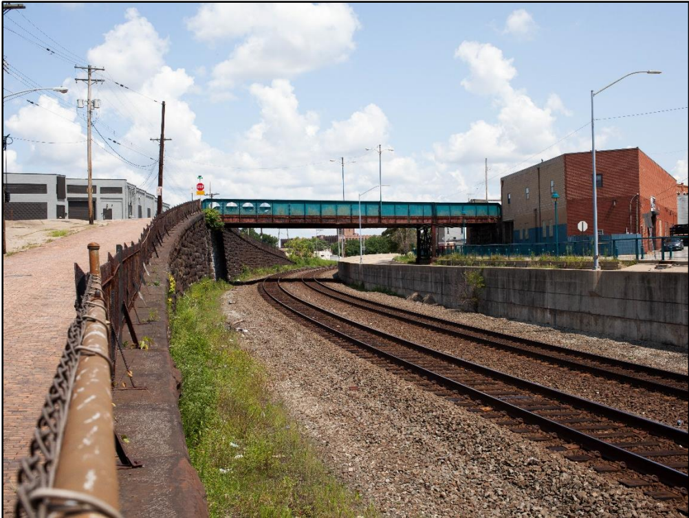
Figure 3-11: Photo of existing tracks under the Washington Avenue Bridge, facing north.
