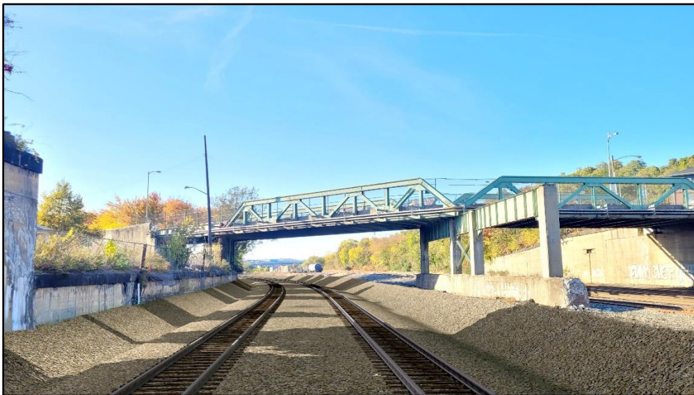
Figure 7-17: Rendering of lowered western-most main line tracks (Alternative 3B) under the Columbus Avenue Bridge, facing northwest.
