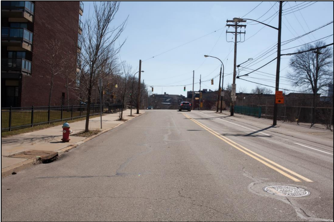
Figure 5-43: Photo of existing W. North Avenue Bridge from Brighton Road, facing southeast.
