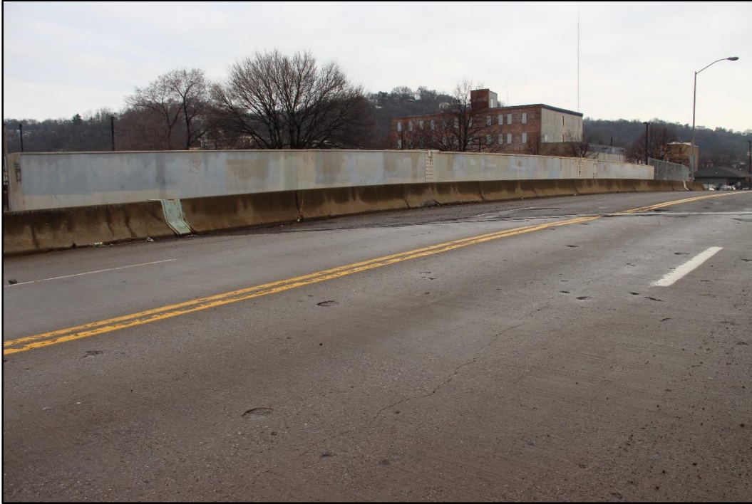
Figure 6-9: Pennsylvania Avenue Bridge showing the deck and southeast girder, facing southwest.
