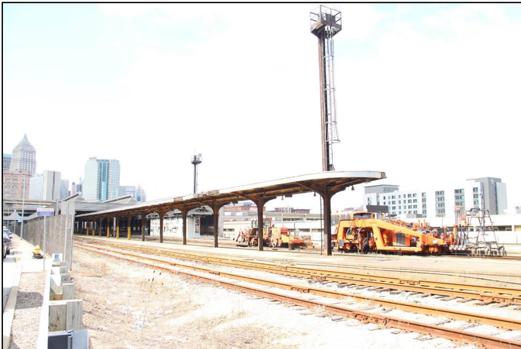
Figure 4-7: View of contributing portion of railyard showing northeast façade of trainshed (1953-59) with umbrella sheds covering Platforms 2 and 3, assistant rail master office, and observation towers (visible in the foreground and background). View from Martin Luther King, Jr. East Busway, facing west.
