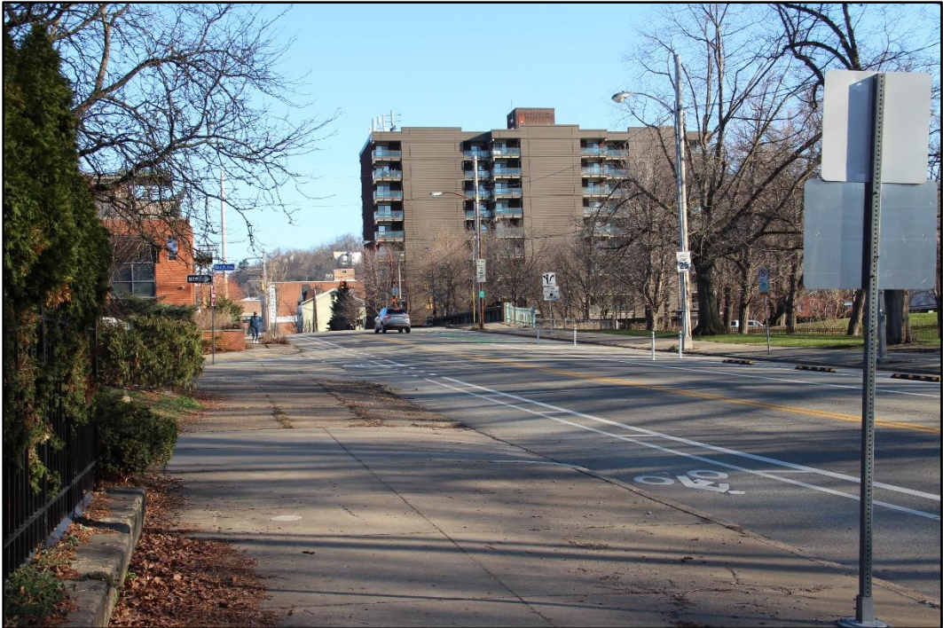
Figure 5-50: View from northeast corner of the Allegheny West Historic District boundary and nearest contributing property at 913 Brighton Road, facing north. The vertical alignment adjustment in the 900 block of Brighton Road would begin approximately 90' to the north.
