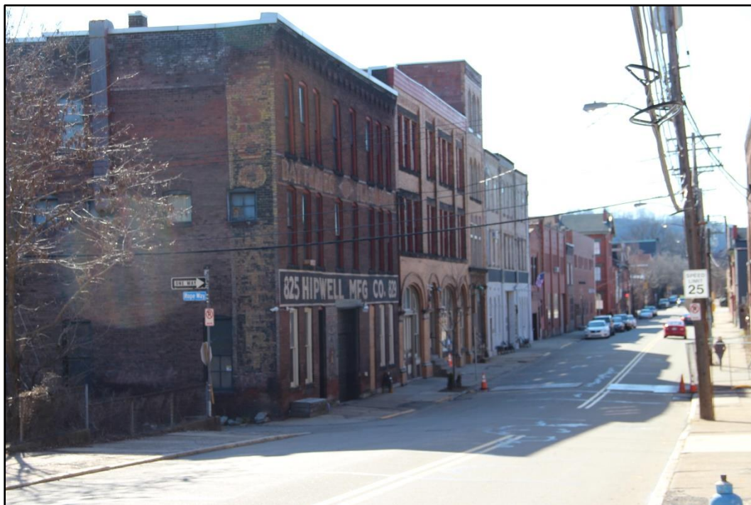
Figure 5-23: South side of the 800 block of W. North Avenue in the Allegheny Second Ward Industrial Historic District from W. North Avenue Bridge, facing southwest.
