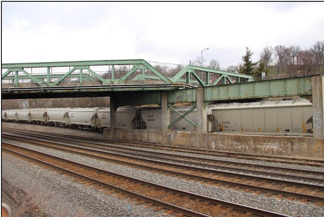
Figure 7-4: Columbus Avenue Bridge showing southeast profile, facing north.
