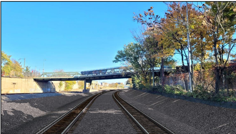
Figure 7-19: Rendering of lowered western-most main line tracks (Alternative 3B) under the Columbus Avenue Bridge, facing southeast.
