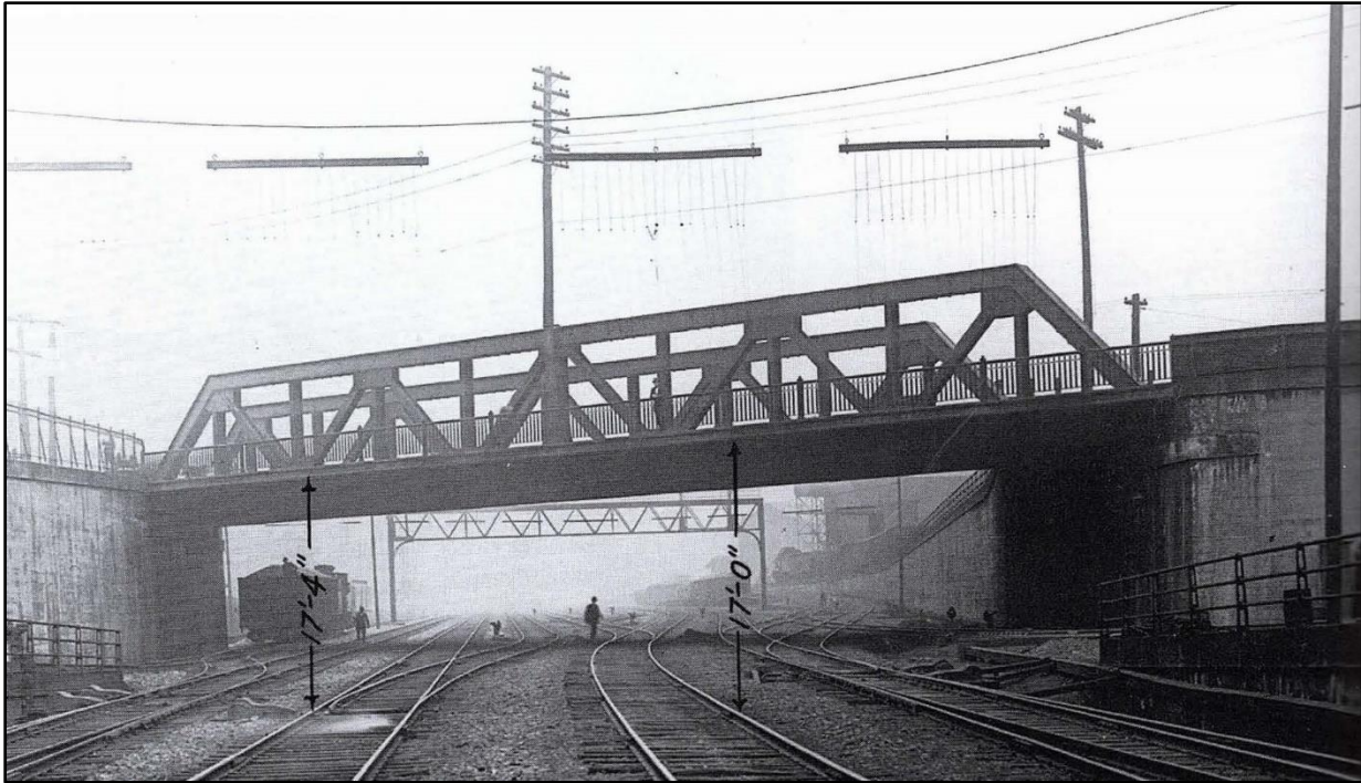
Figure 6-27: Historical photograph dated March 29, 1910, showing the original Warren pony truss bridge carrying Pennsylvania Avenue over the rail corridor, facing northwest.
