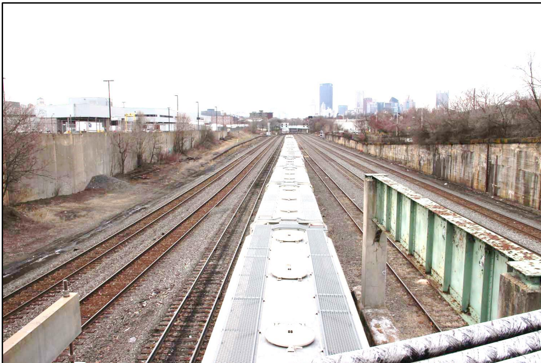
Figure 7-3: View of surveyed segment of rail corridor from center of Columbus Avenue Bridge, facing southeast.
