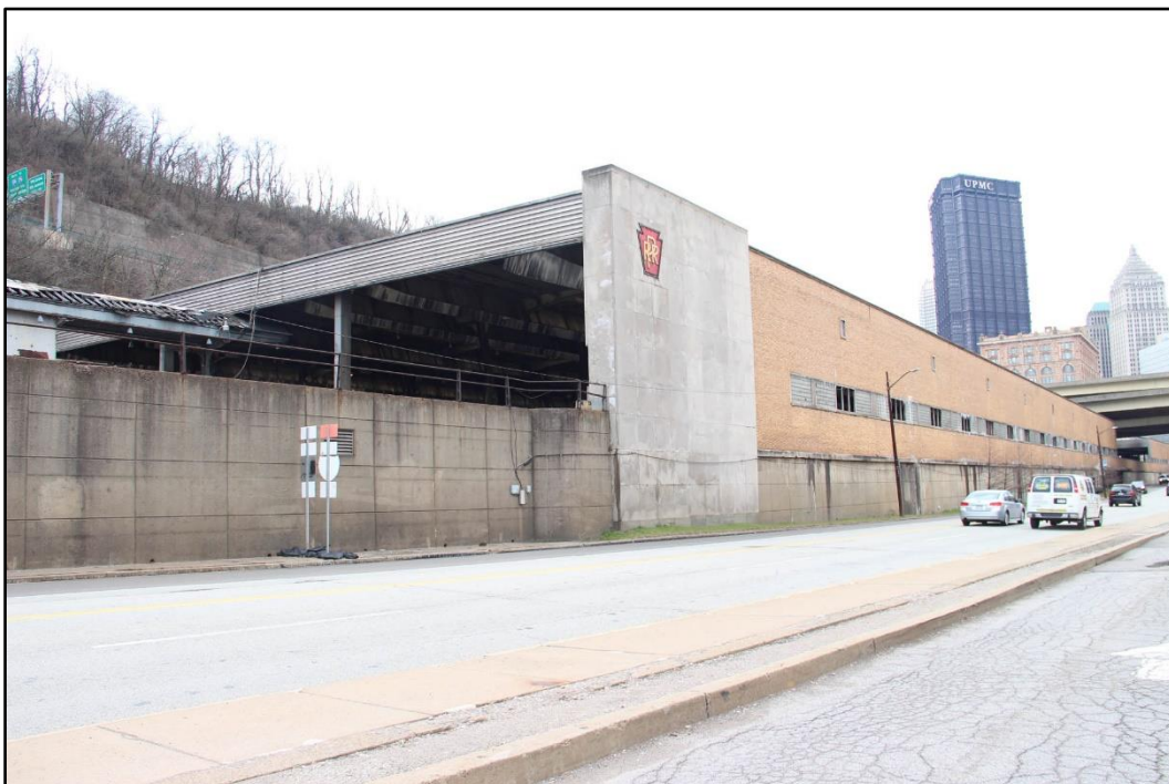
Figure 4-5: Northwest and northeast façades of contributing trainshed (1953-59) showing northeast limestone-clad pylon with terra cotta PRR insignia. View from Liberty Avenue, facing south.
