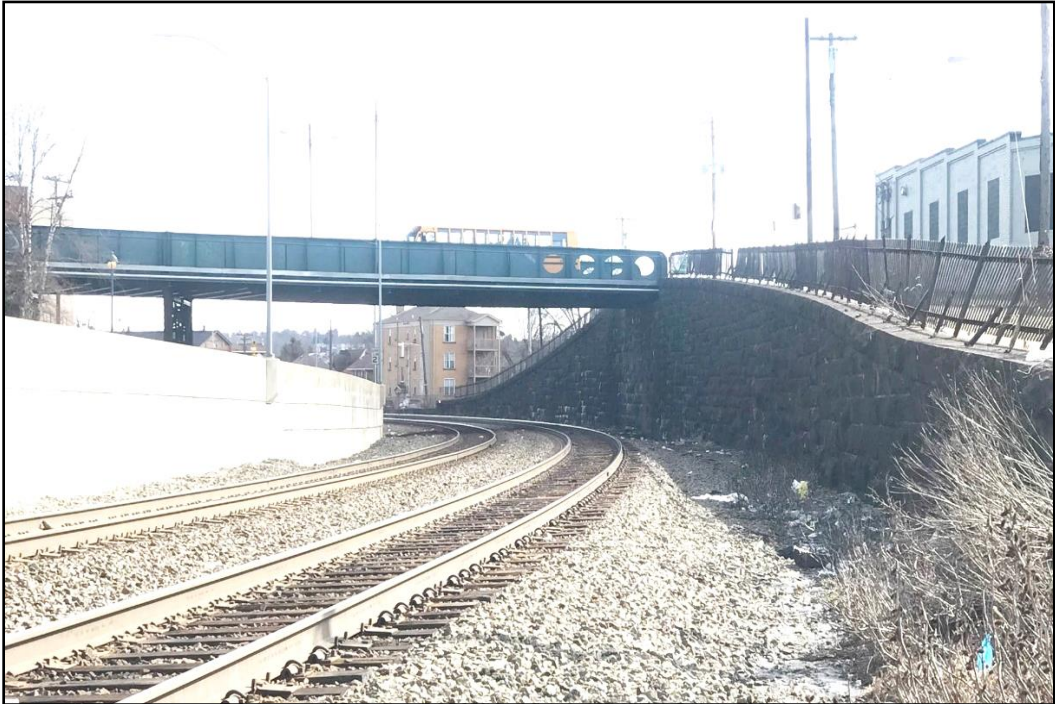
Figure 3-3: Washington Avenue Bridge showing northwest profile, southwest stone abutment and curvilinear retaining wall of the Palmer Street approach ramps, and wrought-iron fencing atop retaining wall, facing south.
