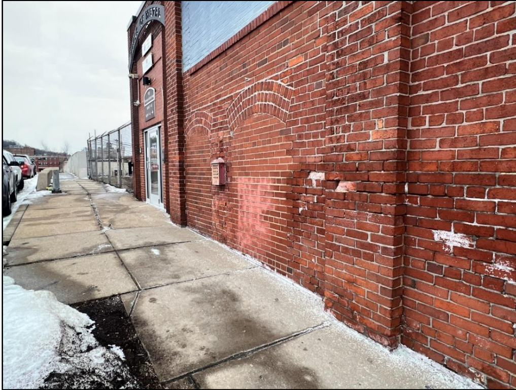
Figure 6-25: Photo of existing sidewalk and entrance to 901 Pennsylvania Avenue, facing northeast.
