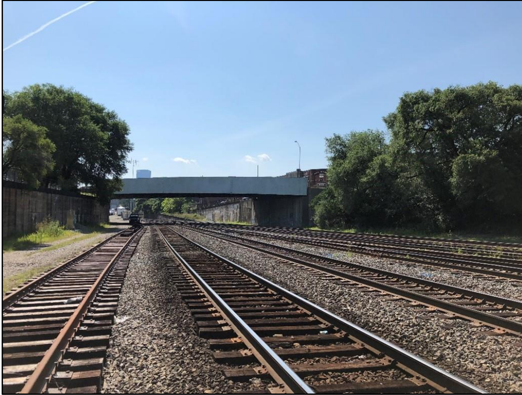
Figure 6-19: Photo of existing Pennsylvania Avenue Bridge from track level, facing southeast.
