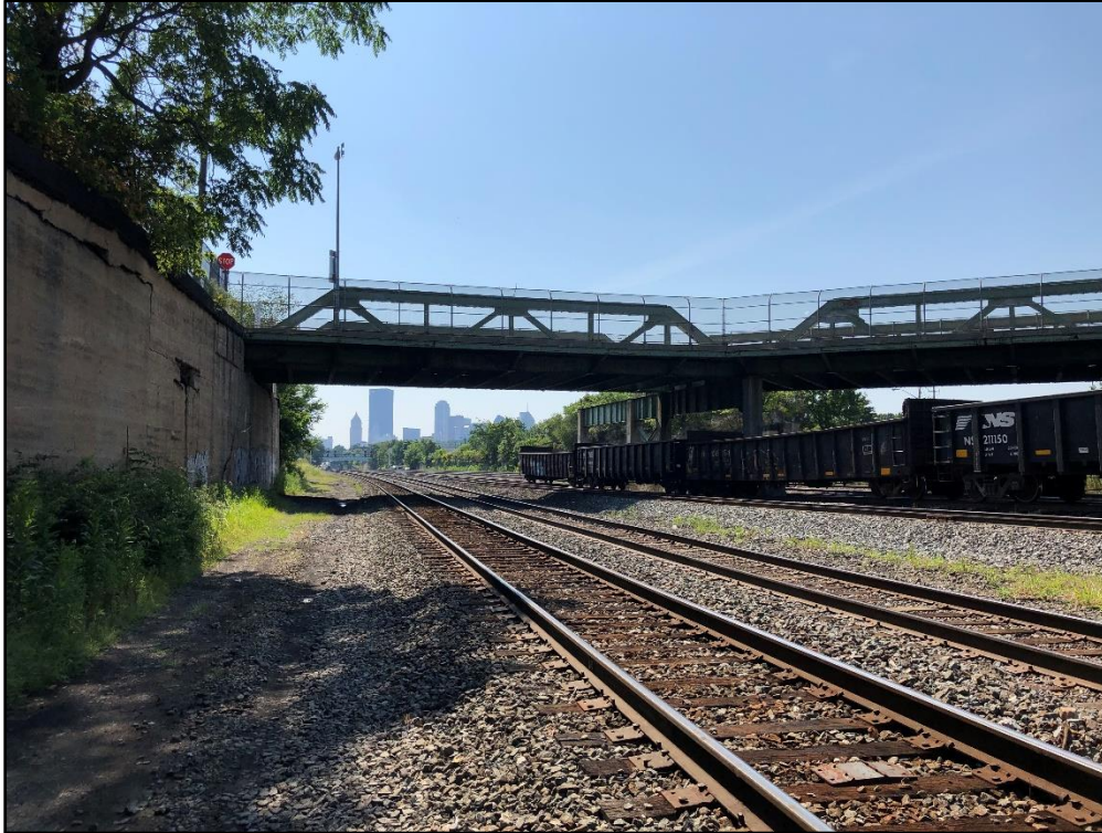
Figure 7-14: Photo of existing eastern-most main line tracks under the Columbus Avenue Bridge, facing southeast.
