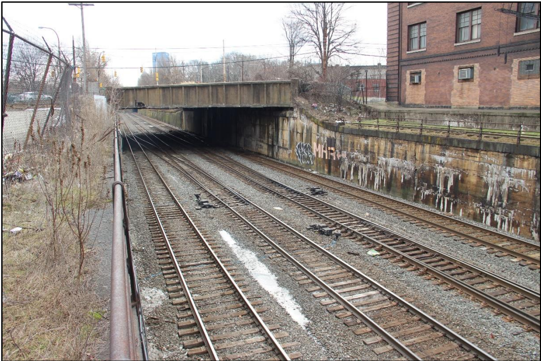
Figure 5-3: View of surveyed segment of rail corridor from the northeast retaining wall showing northwest side of the W. North Avenue Bridge, the southwest concrete and stone retaining walls, and standard railroad safety fencing, facing southeast.
