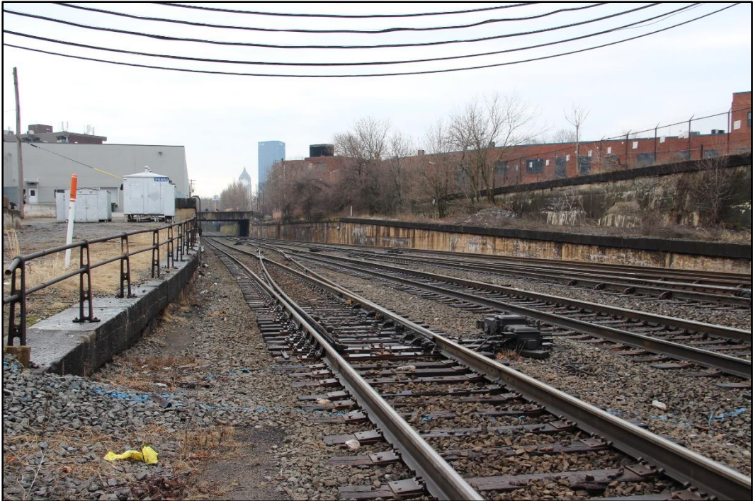
Figure 6-7: Detail of standard railroad safety fencing (left) along edge of ramp to former elevated siding along the northeast side of the corridor, facing southeast.
