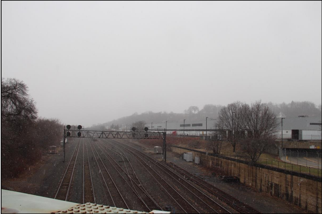
Figure 6-5: Rail corridor from Pennsylvania Avenue Bridge showing northeast concrete retaining wall with stone coping along USPS facility, facing north.
