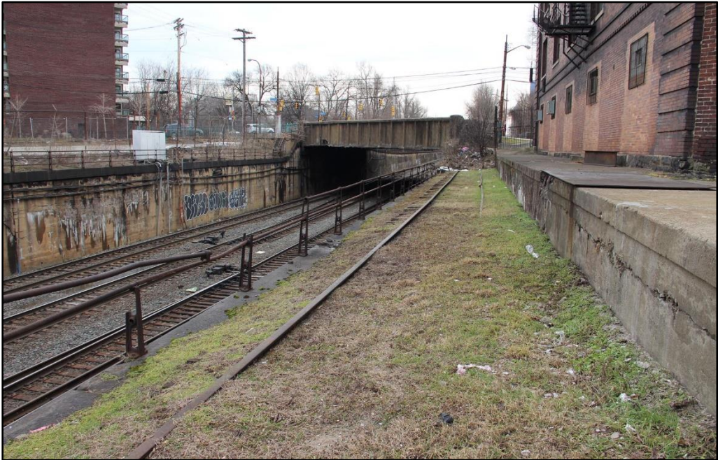
Figure 5-11: View of out-of-service elevated rail siding for the former International Harvester Building along the southwest side of the rail corridor north of the W. North Avenue Bridge, facing southeast.
