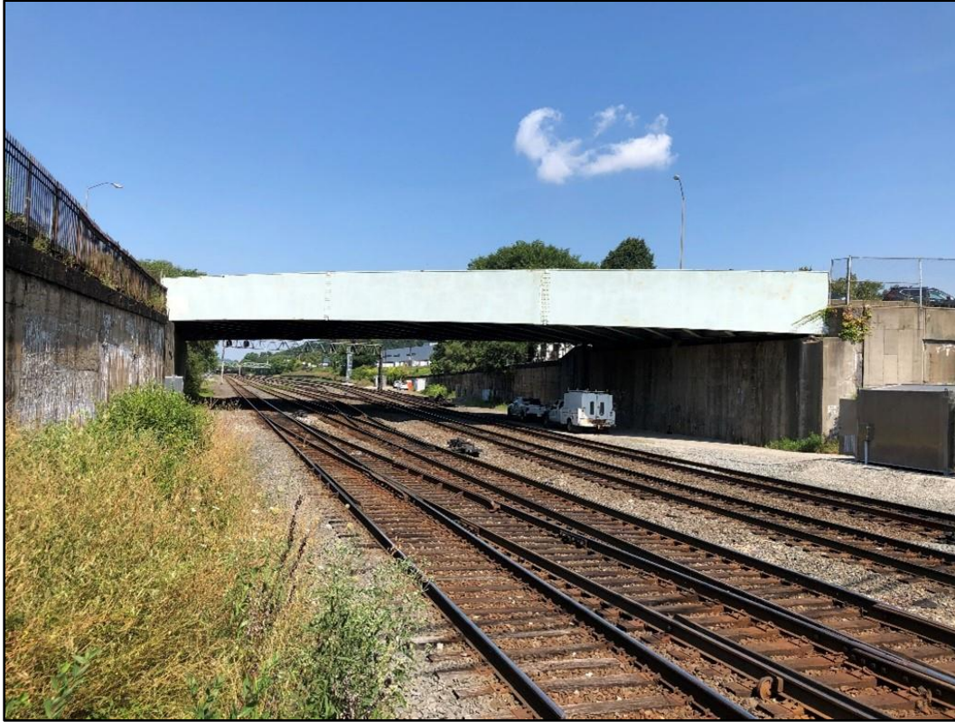
Figure 6-17: Photo of existing Pennsylvania Avenue Bridge from track level, facing northwest.
