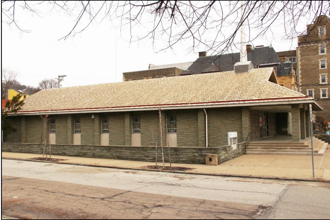
Figure 5-18: West (side) and south (front) façades of 622 W. North Avenue, a non-contributing element of the Mexican War Streets Historic District, facing northeast.
