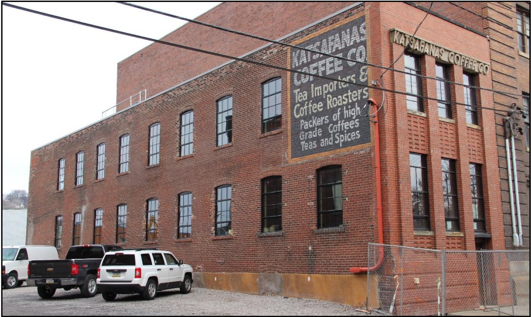
Figure 5-26: West (side) and south (front) façades of the Katsafanas Coffee Company Building, 828 W. North Avenue, a contributing element of the Allegheny Second Ward Industrial Historic District, facing northeast.
