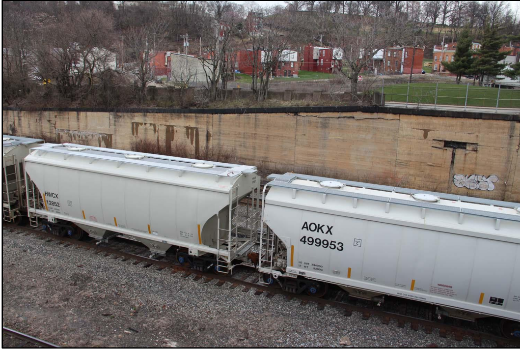
Figure 7-5: Detail of rail corridor showing northeast reinforced concrete retaining wall with stone coping along California Avenue, facing north.
