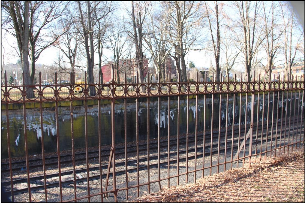
Figure 5-9: Decorative wrought iron fencing atop the stone and concrete retaining walls of the depressed railroad corridor through Allegheny Commons Historic District, facing west.
