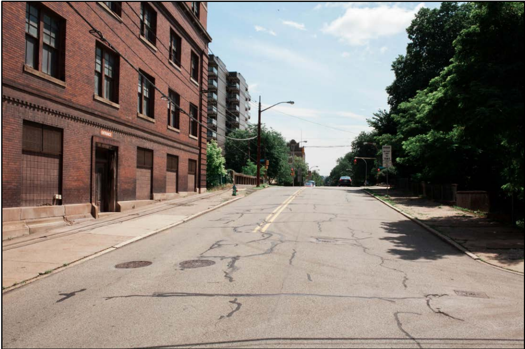
Figure 4-25: Photo of existing W. North Avenue Bridge from W. North Avenue Road, facing northeast.
