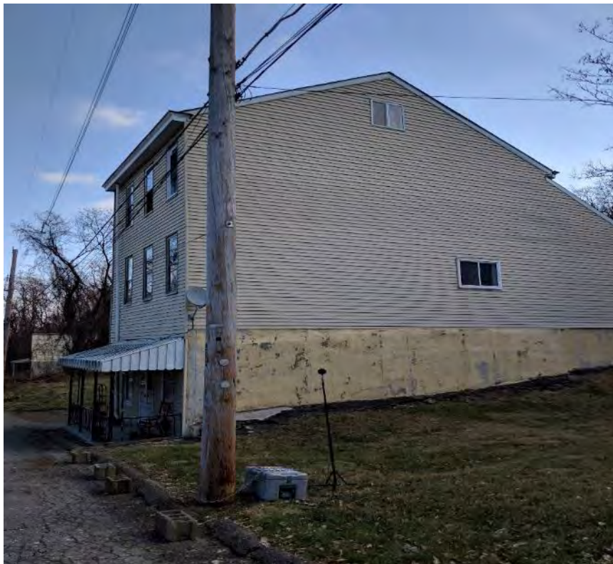
Figure A-10. Site LT-10: 2630 Brereton Street
