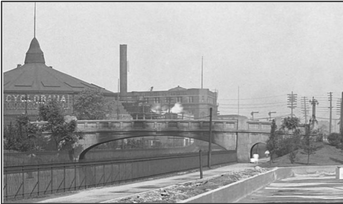
Figure 3-11: Historical photograph dated July 8, 1920, showing the former poured concrete Allegheny Commons Pedestrian Bridge carrying a park path over the rail corridor, facing northwest (University of Pittsburgh).
