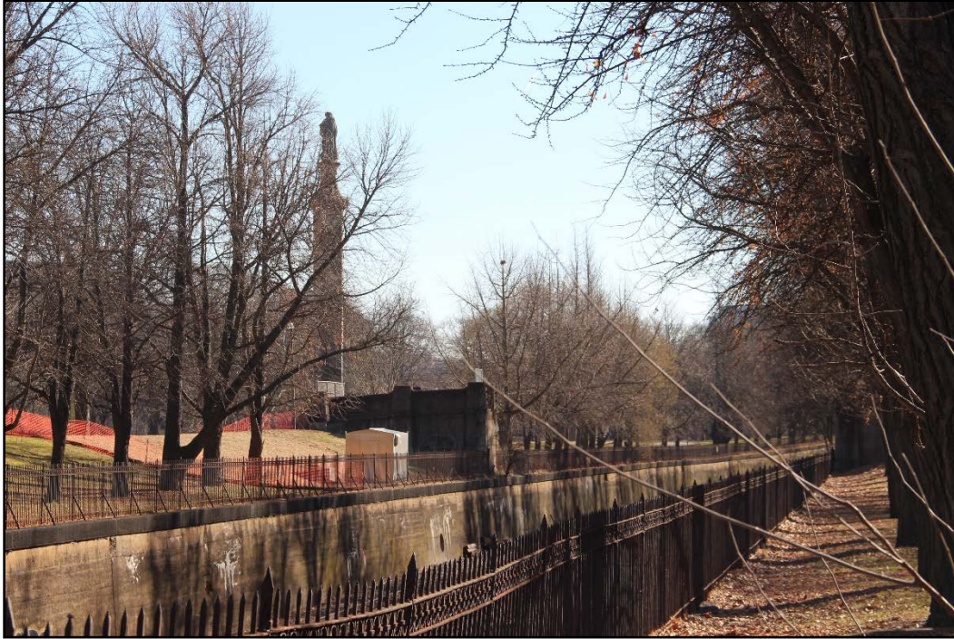
Figure 3-2: Allegheny Commons Pedestrian Bridge Project location, showing the depressed railroad corridor with concrete retaining walls with stone coping and decorative wrought iron fencing, facing southeast.
