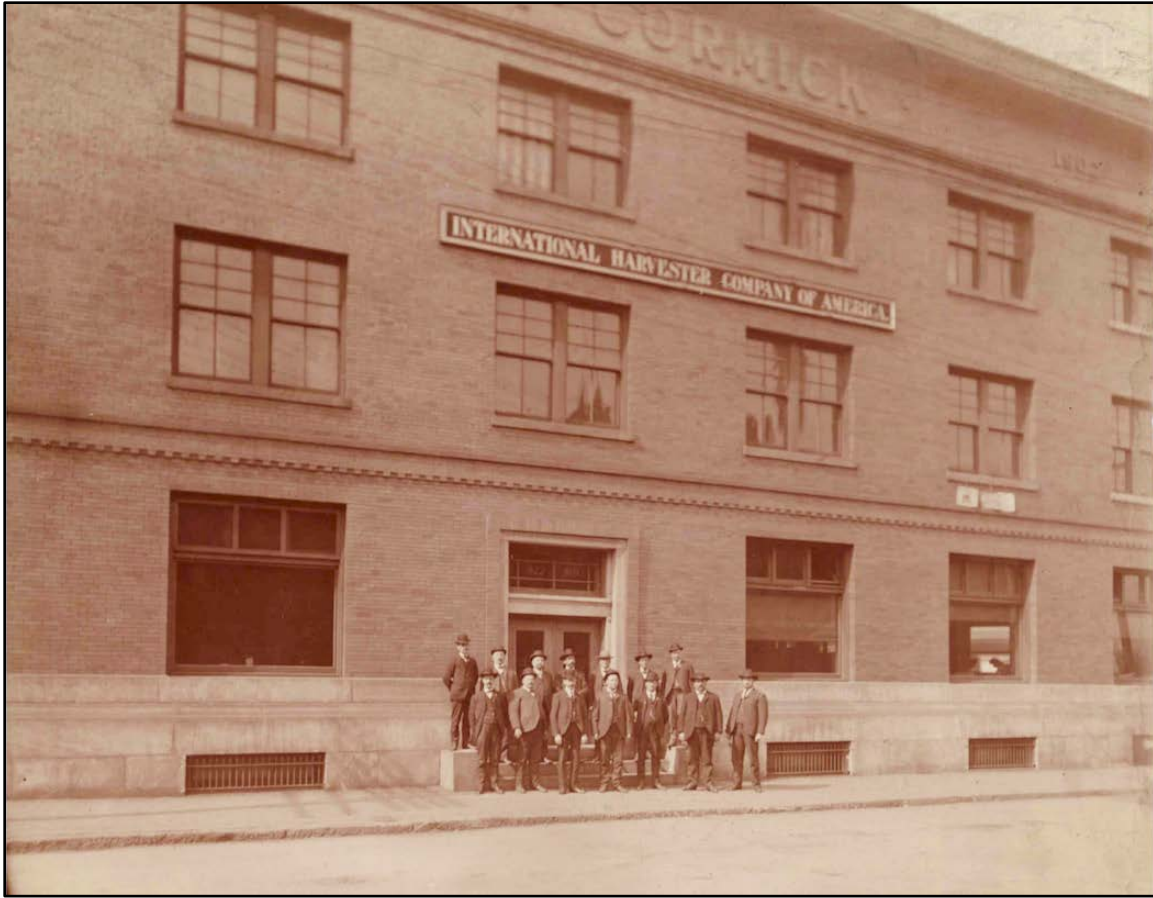
Figure 4-28: View of the International Harvester Building in 1904 showing the limestone foundation/water table and first floor windowsills prior to the grade separation of W. North Avenue and the rail corridor that occurred ca. 1906.
