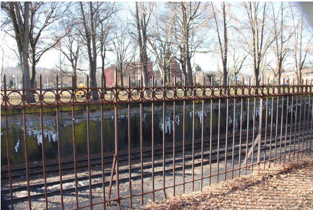
Figure 3-3: Detail of wrought-iron fencing atop retaining wall, facing southwest.
