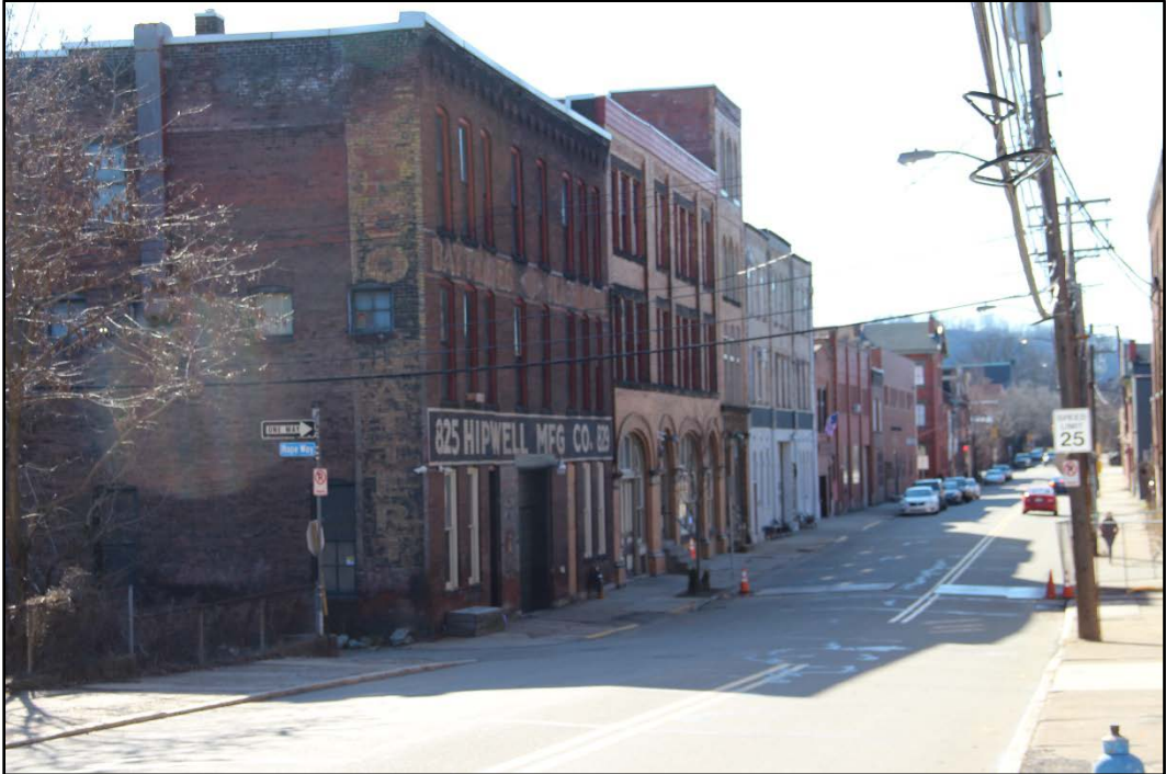
Figure 4-4: South side of the 800 block of W. North Avenue in the Allegheny Second Ward Industrial Historic District from W. North Avenue Bridge, facing southwest.
