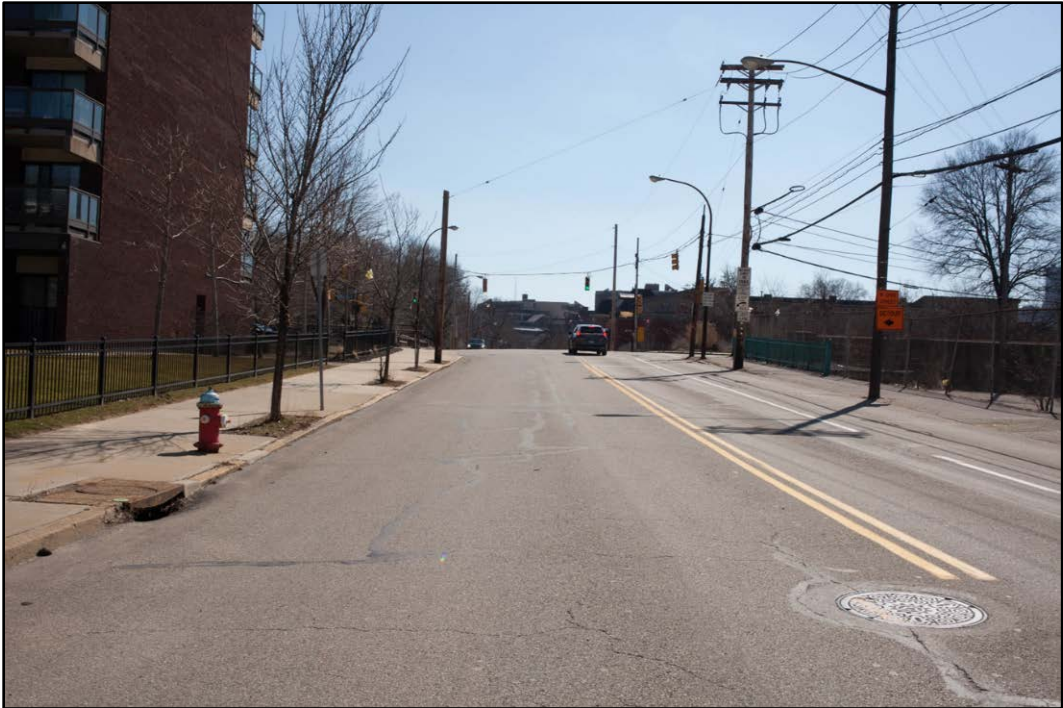
Figure 4-23: Photo of existing W. North Avenue Bridge from Brighton Road, facing southeast.
