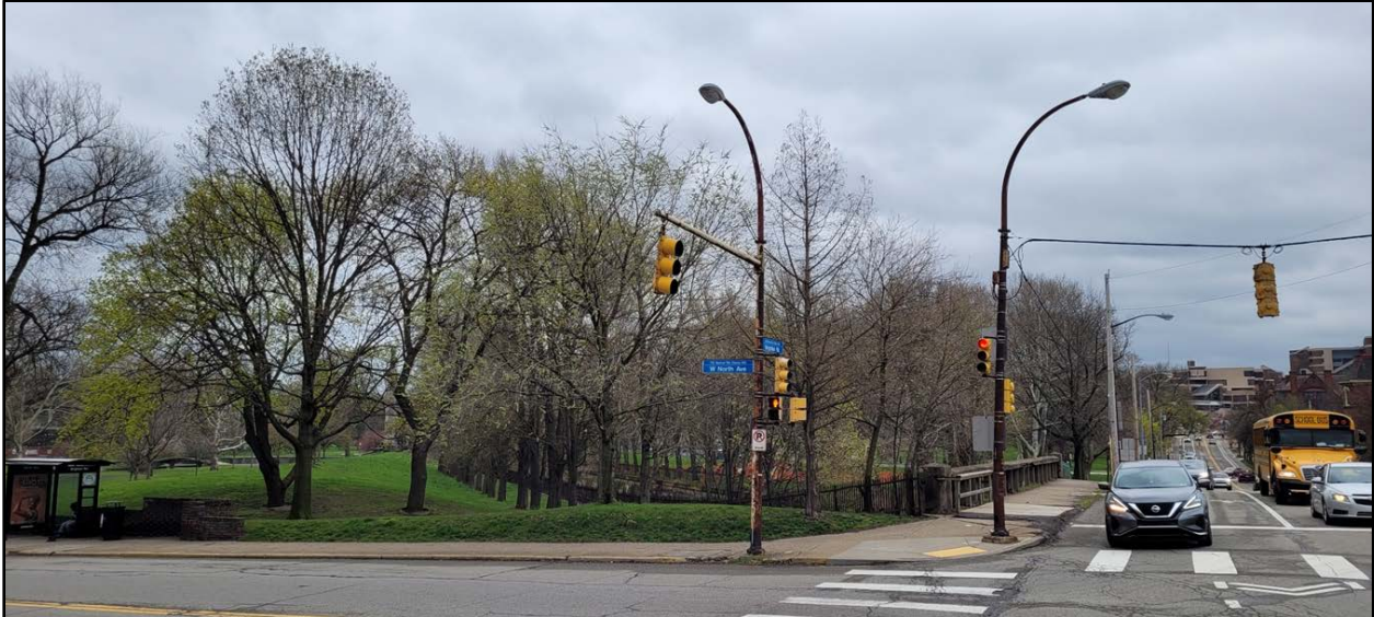
Figure 4-19: Photo of existing W. North Avenue Bridge from street level at the northeast corner of W. North Avenue and Brighton Road street level, facing southeast.
