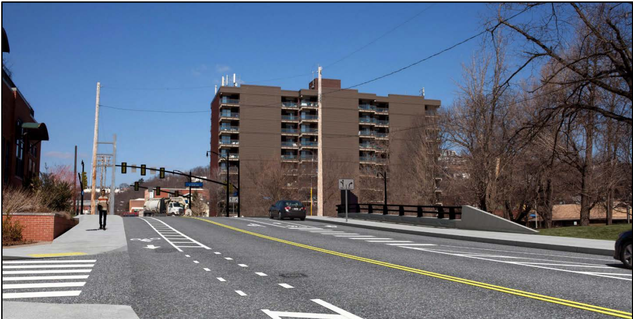
Figure 4-22: Rendering of proposed W. North Avenue Bridge from the southwest corner of Brighton Road and Beech Avenue, facing north. Note the reduced size of the safety barrier transition at right.
